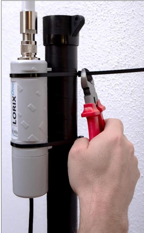
Once the LORIX One well oriented and the cable tie well tight, use a cutting pliers to cut the exceeding plastic part of the cable tie.
